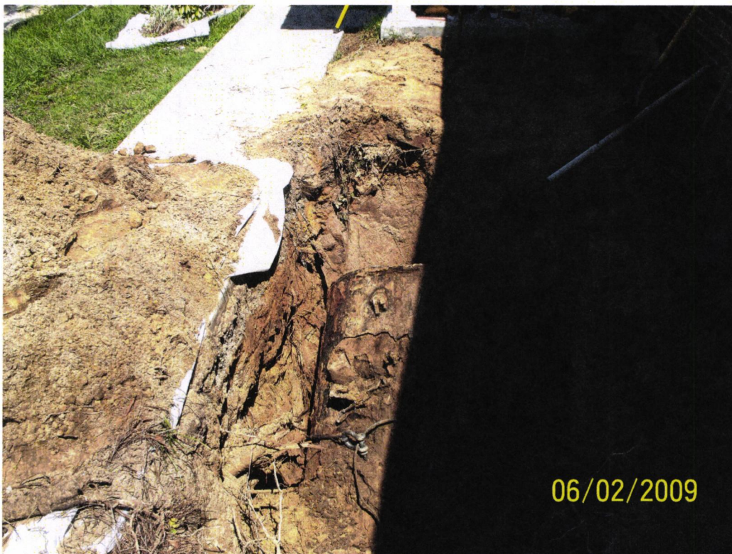
Picture 2: UST 1053Gardenia during removal.
